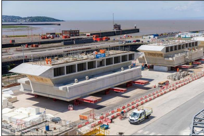
Figure A3-3 -Hinkley Point C's LVSE intake heads are specially designed to reduce the speed at which water is fed into the cooling system
